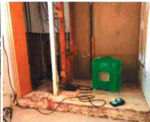
Above Right: Bathroom (Water Heater, Bathtub, Shower wall removed)
