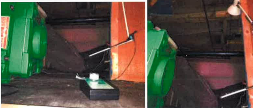
Above Left: Upper level Hallway: Air Sampling Location
