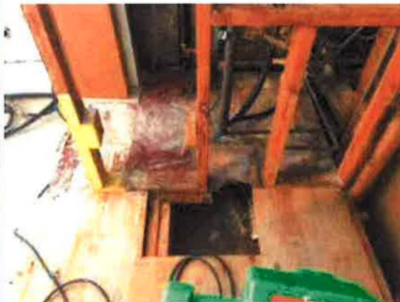
Above Left: Bathroom (Shower wall, Water Heater and Bathtub removed)
