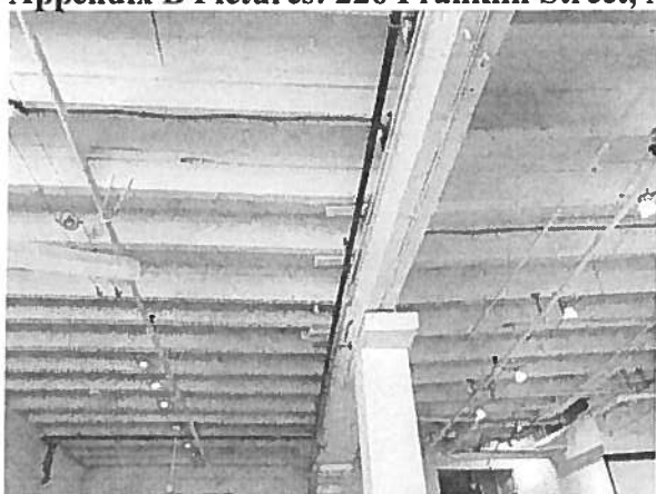
Above left: Living room ceiling with sagging ceiling joists and support beam cracking Above right: Visible mold in studio room 2 west drywall wall
